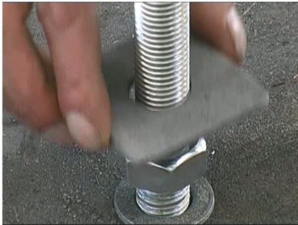
Put the square plates (60x60x5 mm) on top of the bolts
