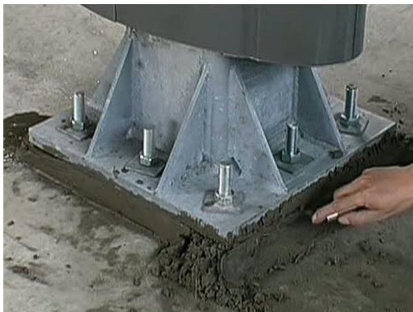
After installation put a shrink free concrete under the base plate!
